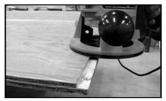
4. If not already done, router the rear edge of the rear sheets of plywood 3/16" down and 1/2" in. If required, also router the sides and/or the front to match the removed plywood.
