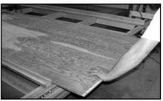
**5.** After routing plywood, slide it in from the rear, screw it down, and replace the rear bumper.
