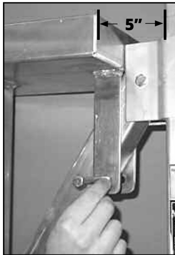
Fig. 10 Attach V-brace Battery Tray
