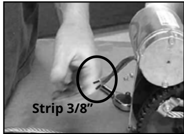
Fig. 7A Strip insulation.
