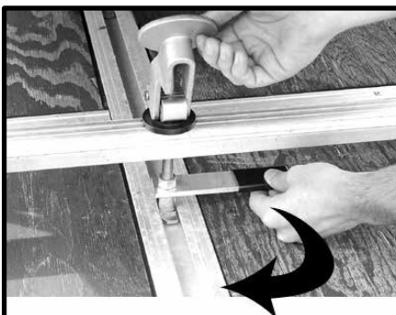
Insert tie down lock and turn 90°
